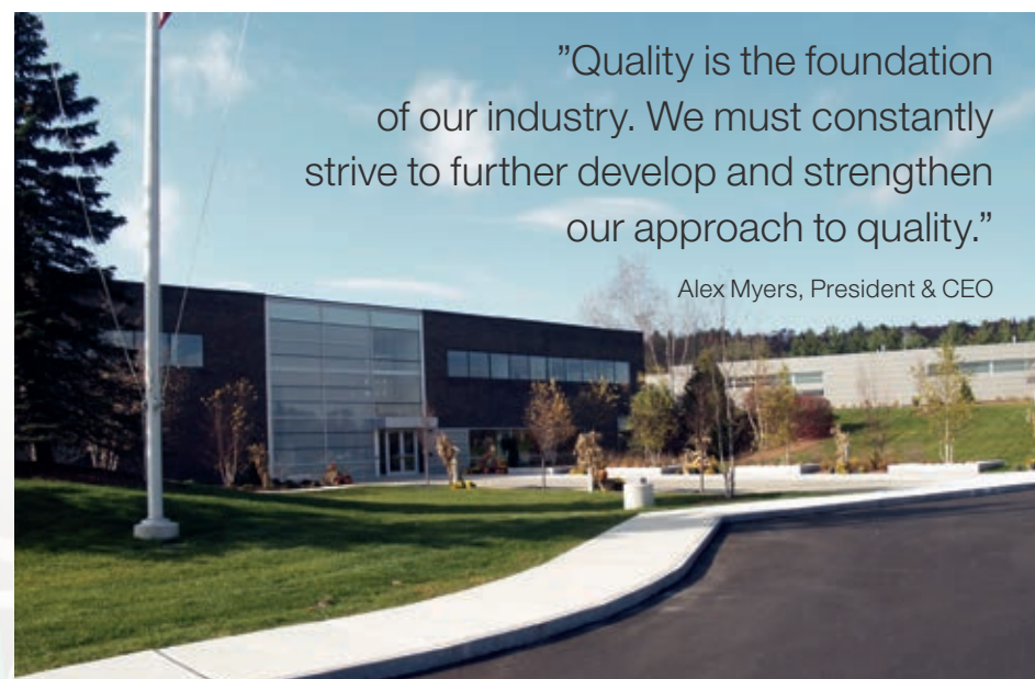
Getinge's new production unit in Merrimack, New Hampshire.
